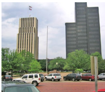
Office towers on each end of the west block of the square leave an awkward empty space between them.
