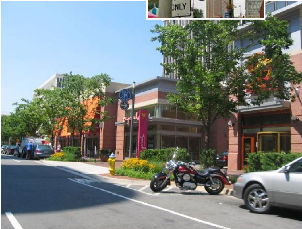
Pedestrian-scale storefronts line taller buildings and a parking garage. Street trees, plantings, awnings, curb bump-outs, on-street parking, simple signs for garage parking, and big and transparent windows all contribute to a pleasant pedestrian environment.
