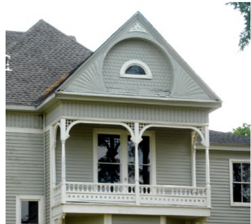
Detailed design guidelines can protect historic architectural features, such as the millwork on this porch.
