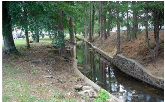
WPA drainage canal
