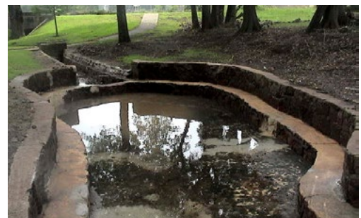
The City should seek education on preservation of its historic infrastructure, including City Park Spring Pond, a Tyler Historic Landmark on West Queen Street.
