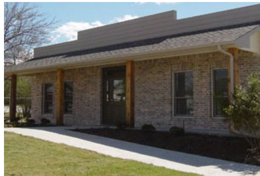
A metal building with a masonry facade in Frisco, TX
