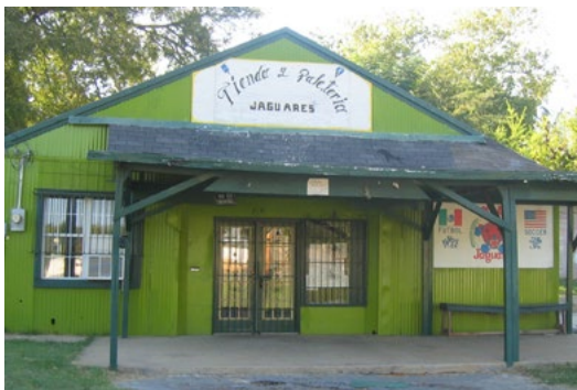
A simple paint scheme can make a metal building more attractive, like this one in Tyler.
