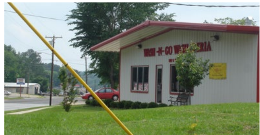
The windows, door, roof overhang and lettering in a simple contrast trim color help this metal building make a better impression.
