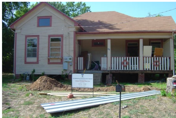
Rehab project funded and managed by the City
