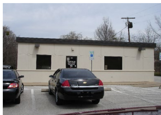
North Tyler police substation
