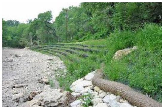
Bioengineering: mechanically-stabilized earth and plantings.
