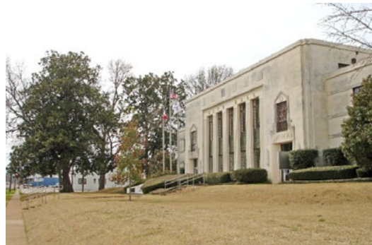
City Hall needs many interior upgrades, but renovations should preserve the building's historic character.
