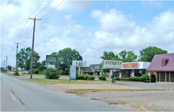
Numerous curb cuts/driveways within short distances of each other create traffic congestion on arterials.
