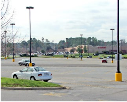
Parking lots often are built to accommodate needs on peak shopping days and remain half-empty the majority of the time.
