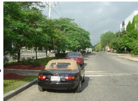
Local access drives separate cars going to businesses along arterials from through traffic.
